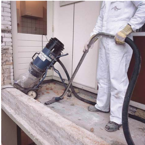
Clean up the dust as soon as possible
